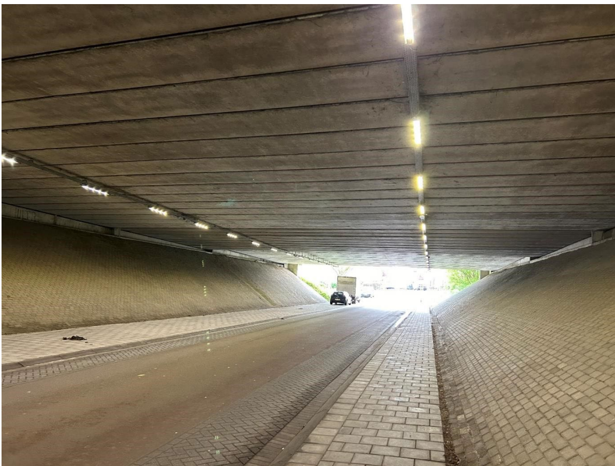
Foto 1: Tunnel Pruiwendijk (A16)
